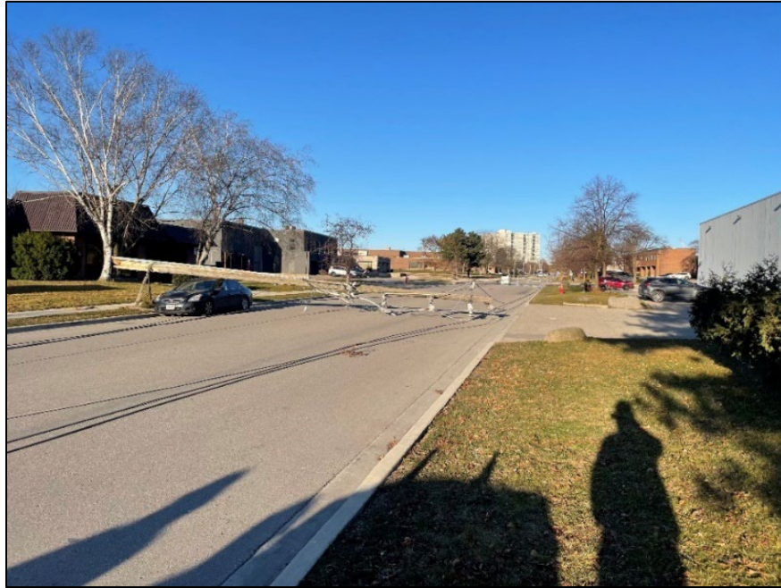
Figure 5.3.2 - 53 Deteriorated and Fallen Wood Pole in Mississauga, December 2024
