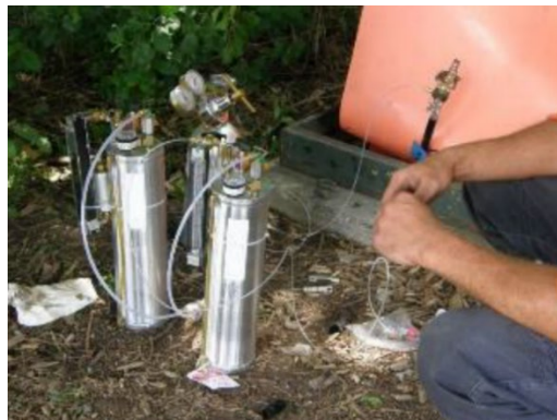
11 Figure 12: Application of cable injection fluid
