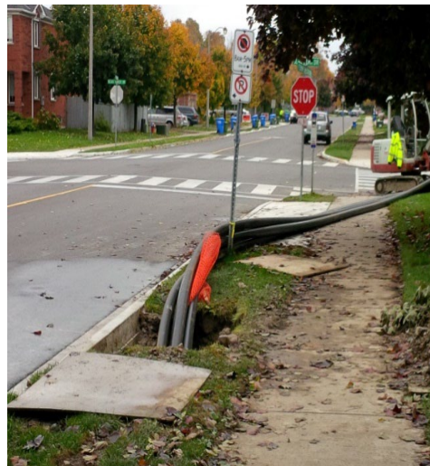
Figure 14: Installation of new cable in duct
