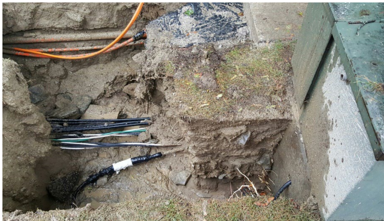
7 Figure 19: Excavated direct-buried cables near pad-mounted transformer base
