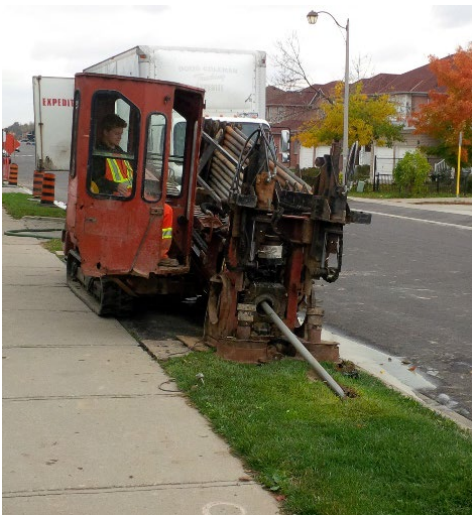
Figure 13: Direction Bore Machine installing new duct for cable replacement
