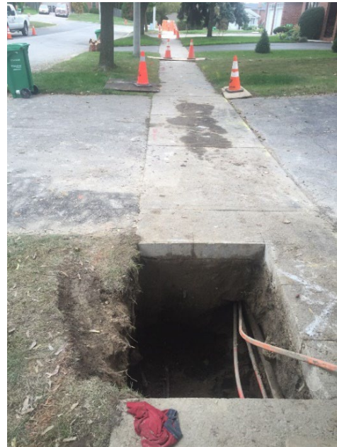
Figure 11: Excavated direct-buried XLPE under a sidewalk
