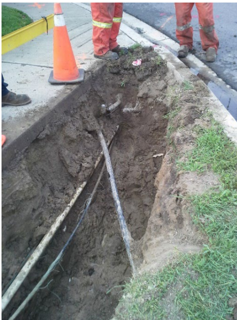
Figure 10: Excavated direct-buried XLPE Cable
